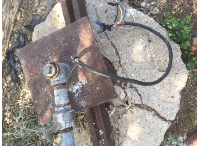
Combs, Lennox Ranch 2 (no test, steel tape too short)
